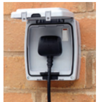
The neoprene seals will not stain the cable.
