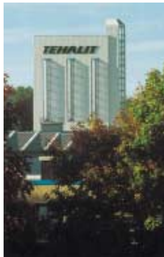
Tehalit headquarters in Heltersberg
