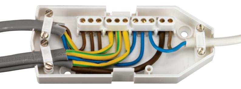
Regulation 526.2 is complied with where the method of connection shall take account of the number and shape of wires forming the conductor. In this junction box solid conductors and flexible conductors can be terminated separately by means of the unique three plate style terminal arrangement.
