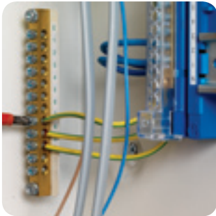
Transparent IP2X shrouds for earth and neutral bars
